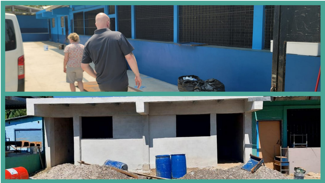
Before and after of the building exterior and the stage.
